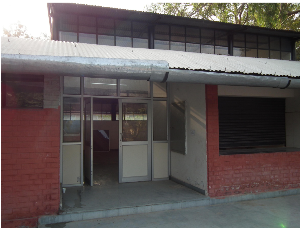
KITCHEN SHED UNDER CONSTRUCTION IN GMSSS Sec-10
