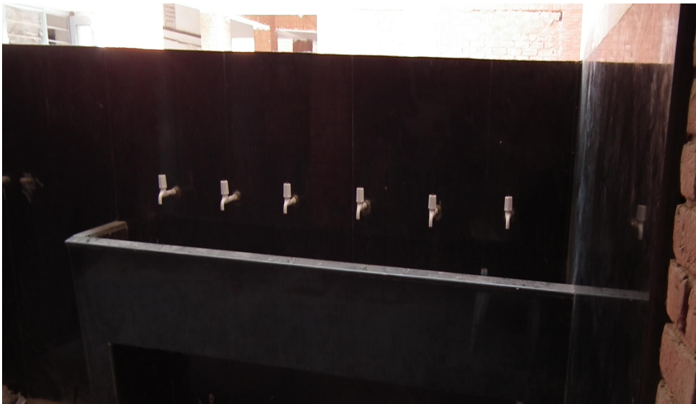
DRINKING WATER ARRANGEMENT IN TWO SCHOOLS (TAPS AND WATERCOOLER)
